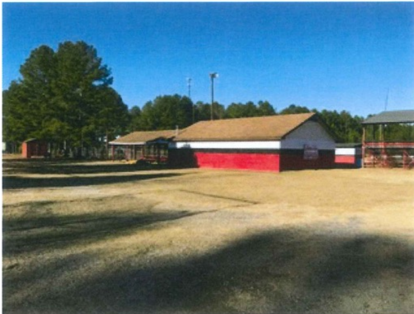
Field 2 buildings with storage shed under tree.
